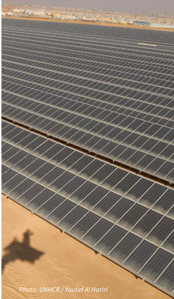
Figure 1 Jordan's Za'atari refugee camp made the switch to clean energy on Monday 13 November, with the inauguration of the largest solar power plant ever built in a refugee setting.
